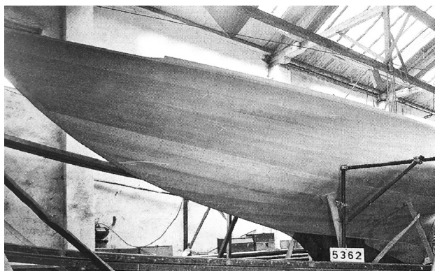
The planks of #60 are now being faired, and high spots requiring further attention have been marked with chalk.
