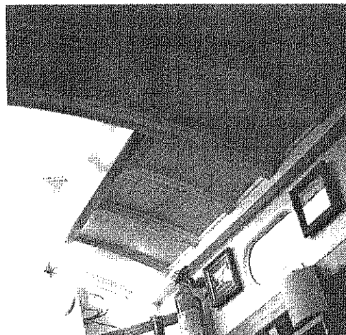
Although a little difficult to see, Yankee's overhead shows coffered paneling that conceals 1/2" foam insulation throughout cabin
